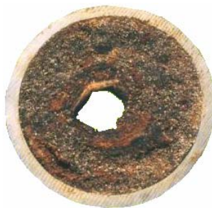
Figure 12 Pipeline petroleum transport plugging due to wax and other heavy organics depositions (see online version for colours)
